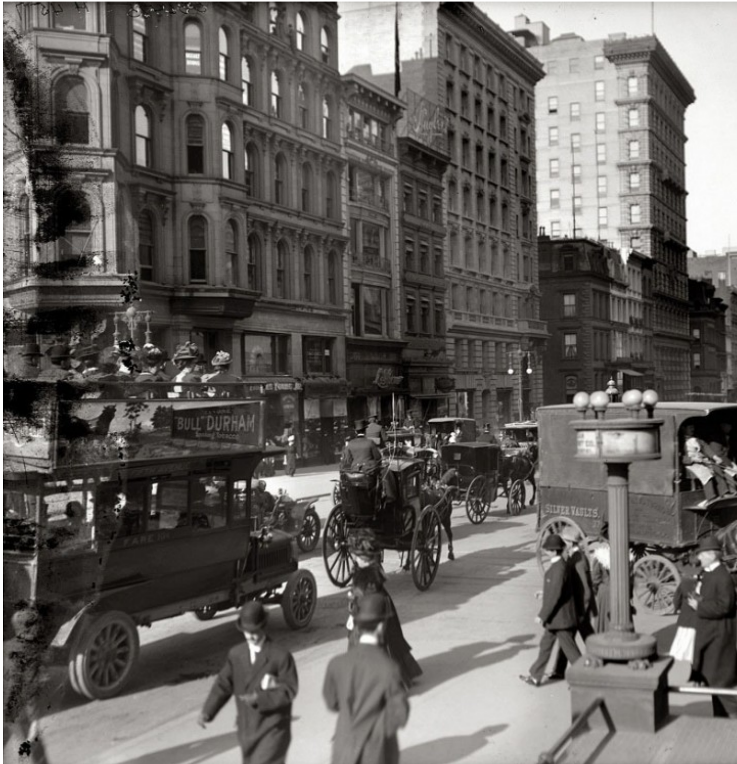
Corner of Fifth Avenue and 42nd Street , New York , 1910.
